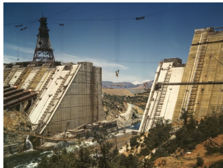
Shasta Dam under construction in June 1942
