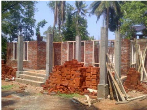
House construction using bricks in Kerala, India
