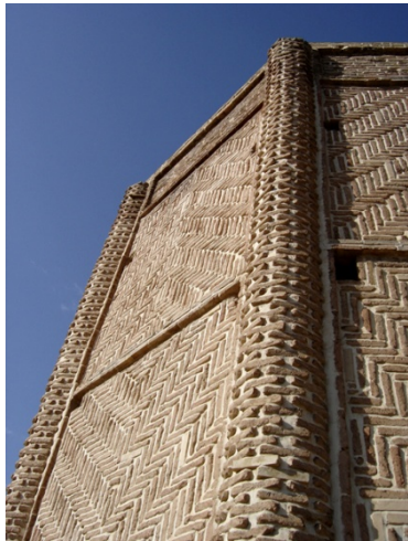
The brickwork of Shebeli Tower in Iran displays 12th-century craftsmanship
