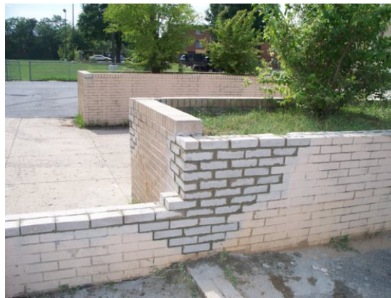
Masonry repair work done to a brick wall
