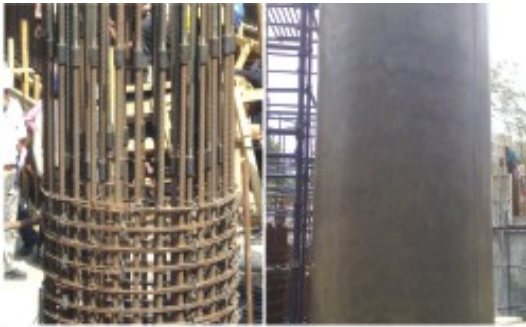
Figure 1: SCC Column (a) Reinforcement couplers (b) Smooth Surface of SCC
