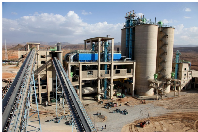
The National Cement Share Company of Ethiopia's new plant in Dire Dawa
