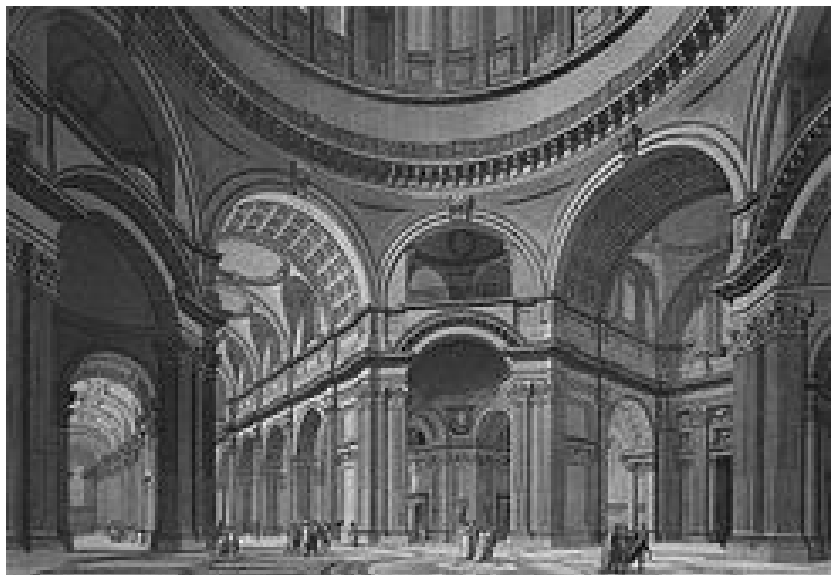
Engraving by Thomas Molton (1792) of the space beneath the dome which reveals how Wren succeeded in giving an impression of eight equal arches.
