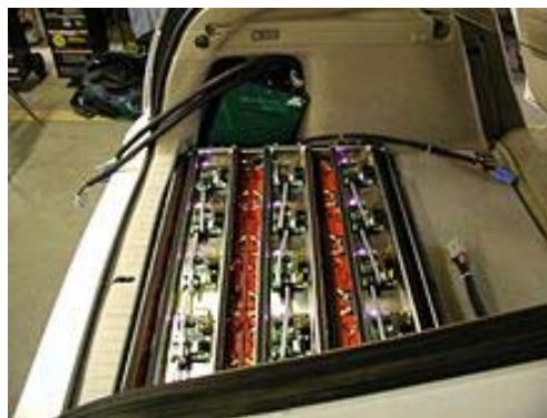
15 lead-acid batteries, PFC charger, and regulators installed into WhiteBird, a PHEV-10 conversion of a Toyota Prius
