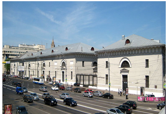
Former Foods Warehouse
