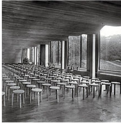
▣ Auditorium of the Viipuri Municipal Library in the 1930s.
